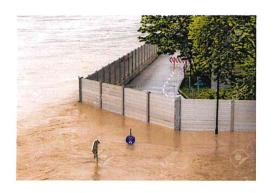
An alternative to permanent walls is a structure or barrier that is put in place in the event of a flood or raises automatically as the water level rises. These can involve a lot of labour and don't actually stop the flooding, but can be very effective in protecting properties in the short-term.
